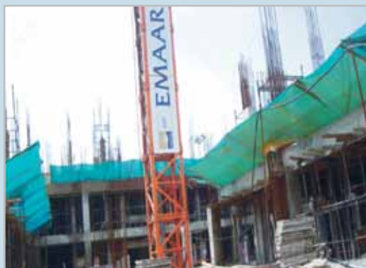
Figure 4 Safety nets at construction site
