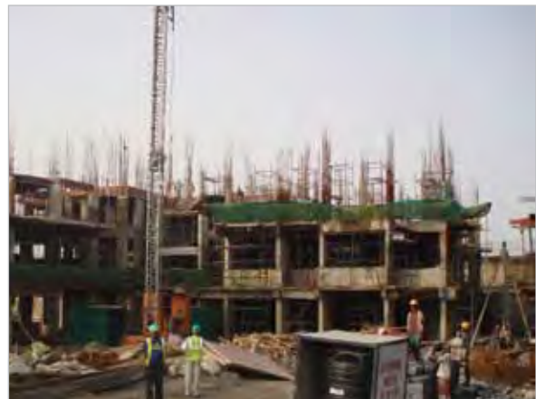
Figure 3 Safety measures in construction site
