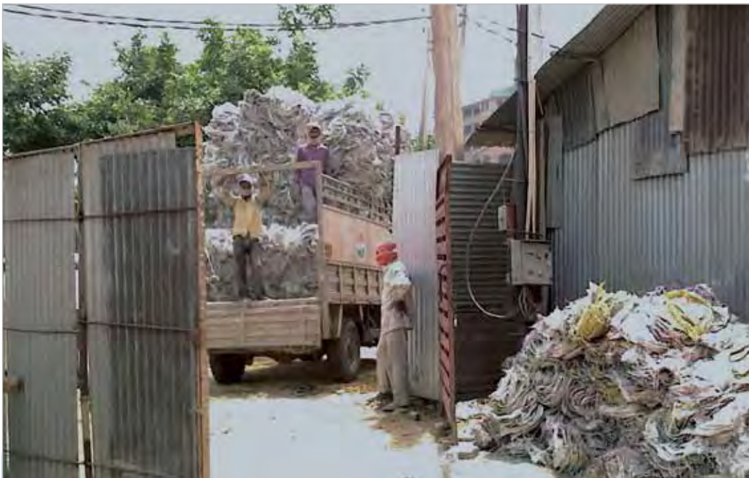
Figure 8 Construction waste disposal
