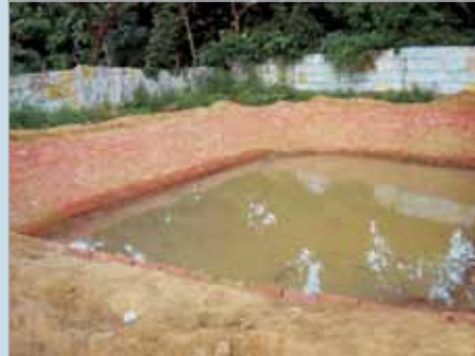
Figure 10 Sedimentation tank
