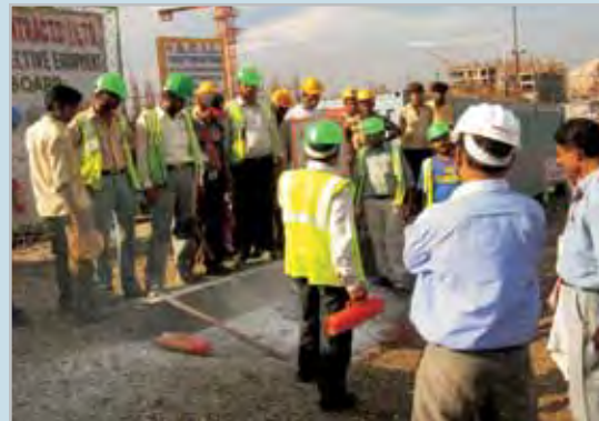
Figure 3 Safety wears during construction
