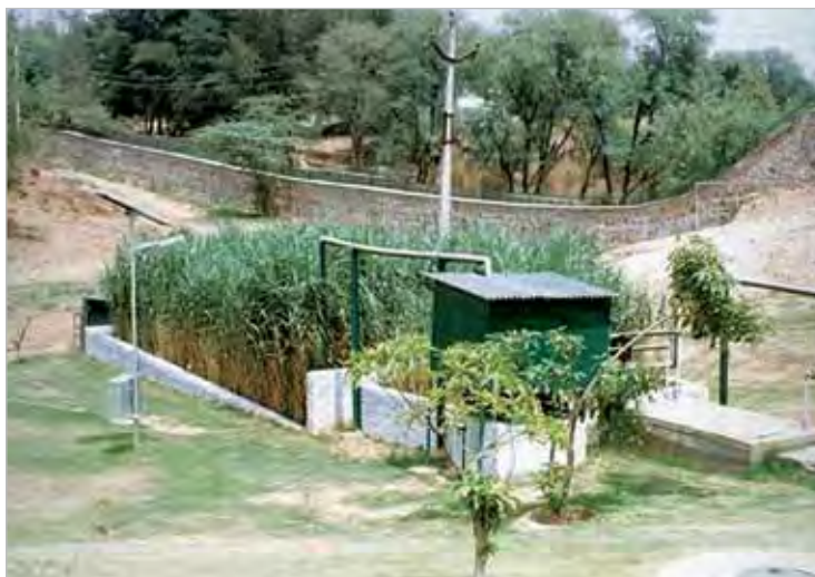
Figure 7 Root zone system for waste water treatment
